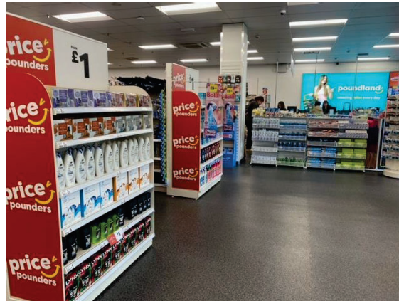
New flooring Internal signage upgraded Replace / upgrade lighting
